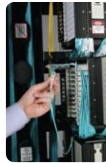
Fiber Termination Block
